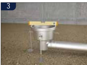
**UK** Bend out the anchor tangs at 90° to the drain. Adjust the drain to the right height and make sure it is level. Fix the drain to make sure that it will not float up during casting.
